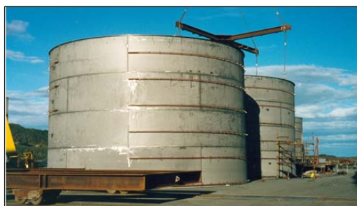
Figure 8. A stainless steel storage tank in the course of erection.
